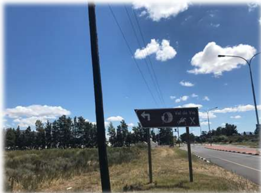
FIGURE 4 VIEW OF MR201, PHOTO TAKEN IN A NORTHERN DIRECTION
